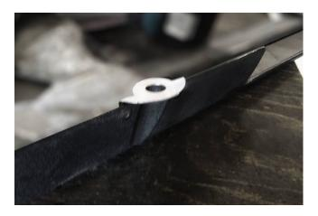
When the angle is correct, hold the sheet and drill the first rivet hole in the bottom of the panel. Deburr a little with the cutter knife and rivet the first rivet. The hole diameter for 3.2mm rivets should be 3.5mm.
